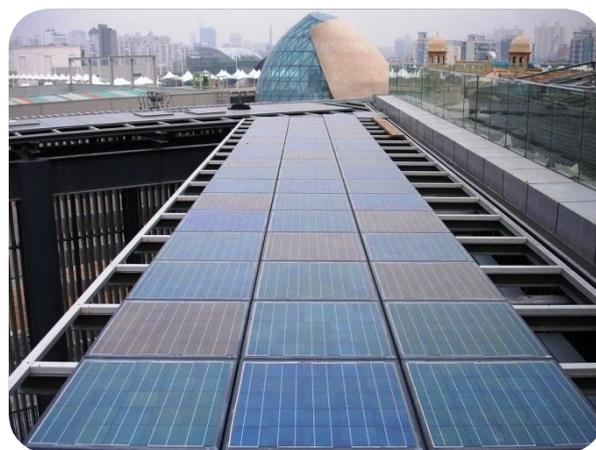
*The supporting structure for LOF color PV panel has been installed. The color PV system will be completed by 2009.*
